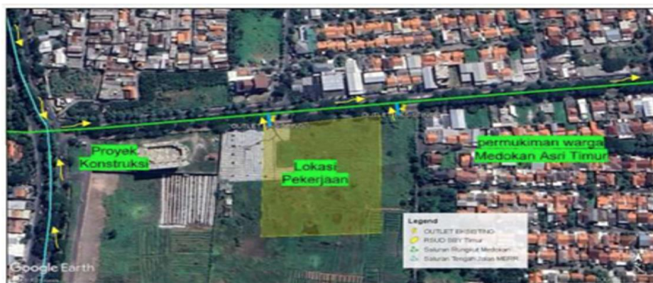
Figure 2. Existing Drainage System of the Work Site Source: Field Survey Results, 2023
